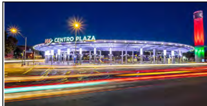
Centro Plaza Transit Center, VIA Metro Transit
