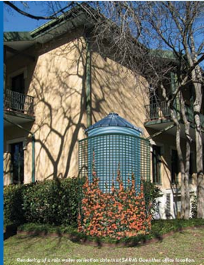
Rendering of a rain water collection cistern at SARA's Guenther office location.
