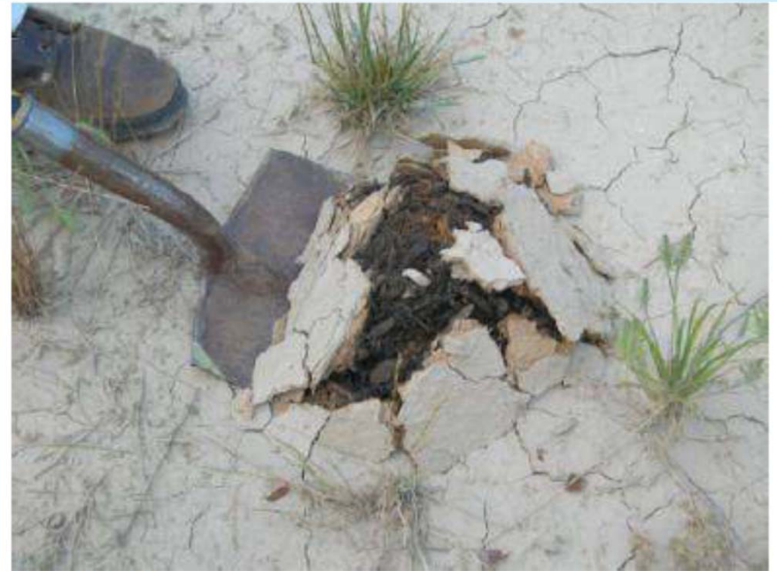
Figure 4-6. Bioretention area clogged with sediment.
