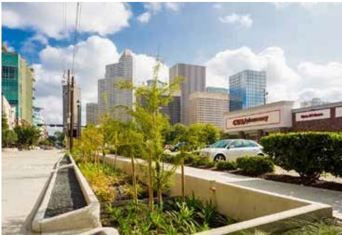
Bagby Street bioretention
