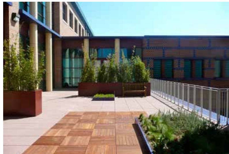
Federal Reserve Bank green roof
