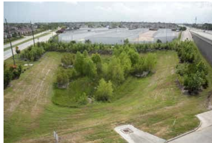
Westpark Tollway bioretention
