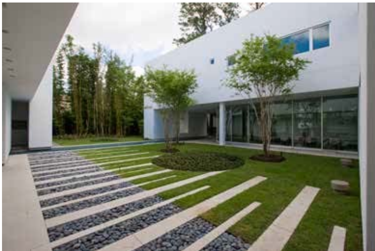
Inverness Residence permeable paving
