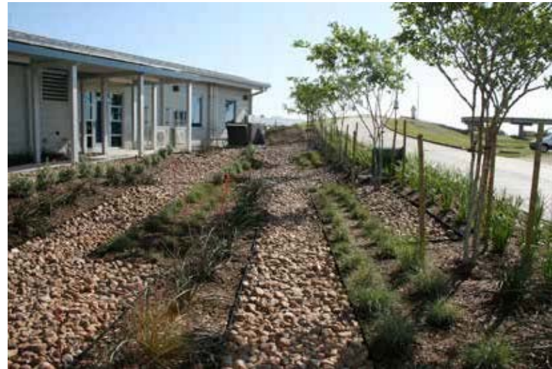
IAH Control Bldg. bioretention
