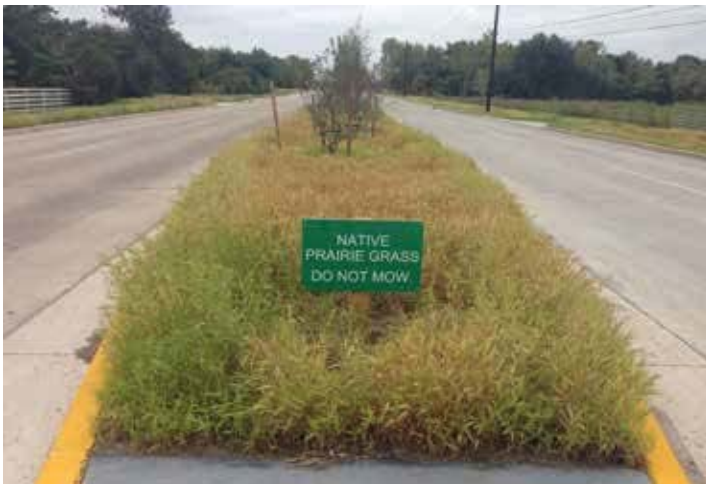
North Main St., Baytown vegetated swale
