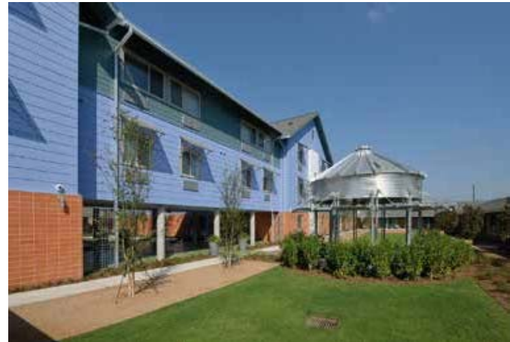
Sakowitz SRO rainwater harvesting
