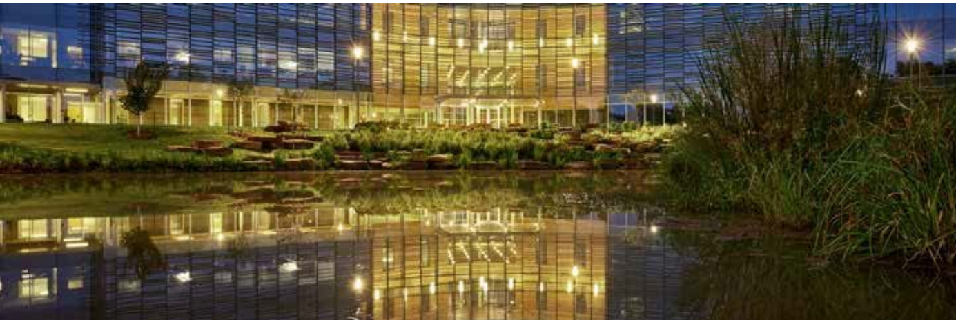
Wildwood Corporate Centre bioretention
