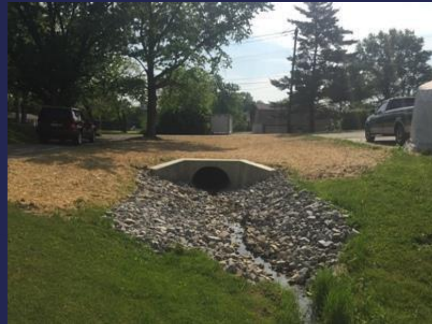
Storm Drain outfall protection with geo-pavers (ArmorLoc) & rip rap
