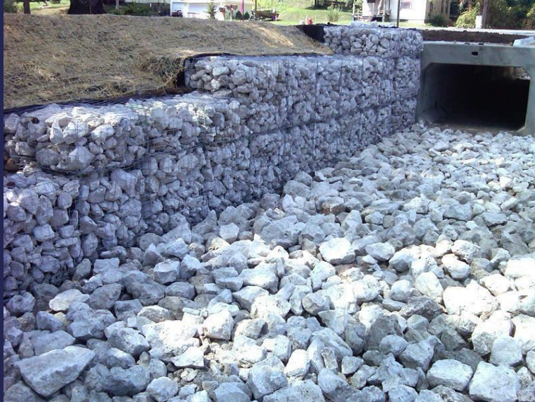
Slope protection at box culvert entrance
