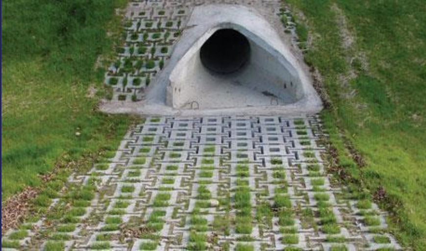
Storm Drain outfall protection with geo-pavers (ArmorLoc) & rip rap
