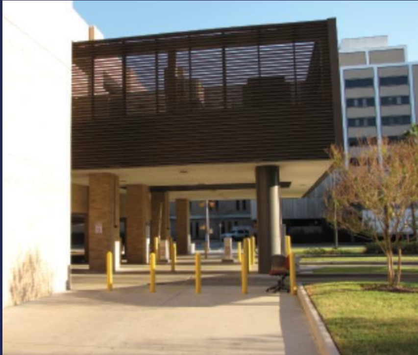
Emergency generator elevated above flood levels at the University of Texas Medical Branch, Hurricane Ike (Galveston, TX, 2008).
