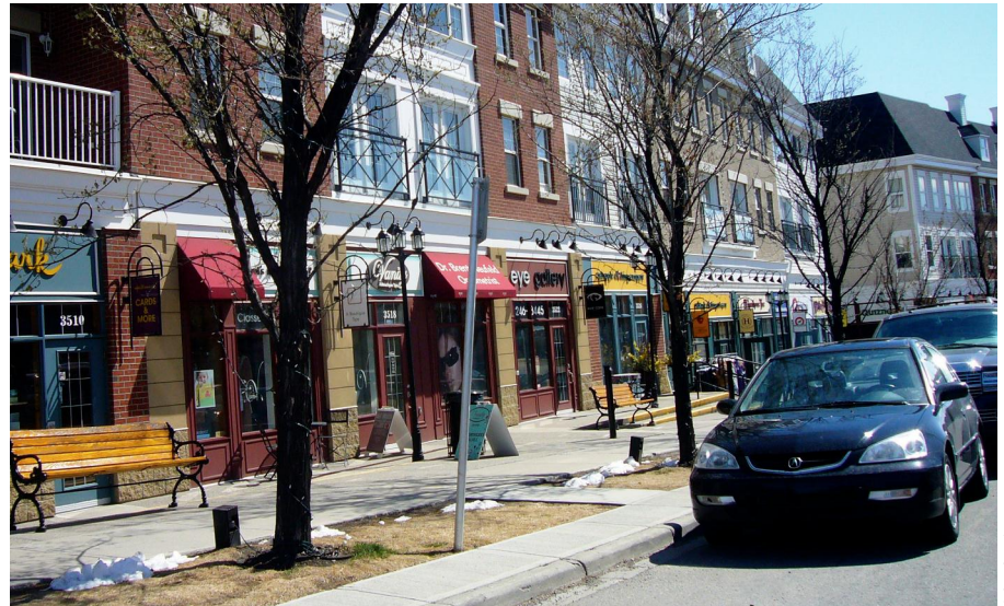
Mixed use with approximately 50 units to the acre. Calgary, AB.
