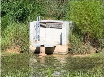
Figure 24: Outfall structure at Houston Botanic Garden Stormwater wetland at low water level. showing clean out ladder.
