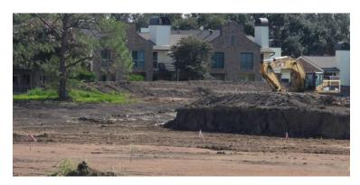
*Figure 19: Photo depicts construction at Exploration Green note the grade stakes in the foreground. Photo courtesy of Jason Miles.*
