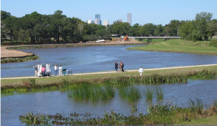
Mason Park Stormwater Wetland along Brays Bayou, Houston, Texas
