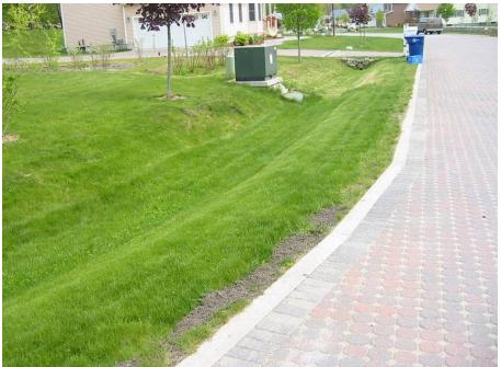
**Swale** – This wide, flat bottomed channel will meander through the park directing water and reducing sheet flow. The grassy bottom of the
