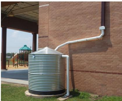
**Rainwater Harvesting** - The roof of the park pavilion is an impervious surface so when it rains the stormwater flows off. This water will be captured and held in a cistern or tank. Between rain storms, this water will be used to water habitat landscapes. Capturing and holding the water keeps it from running, instead when it is used to irrigate on dry days, the water can soak into the ground where organisms in the soil can break down pollutants into harmless compounds.
